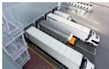
Gates, Doors and Loading Docks
